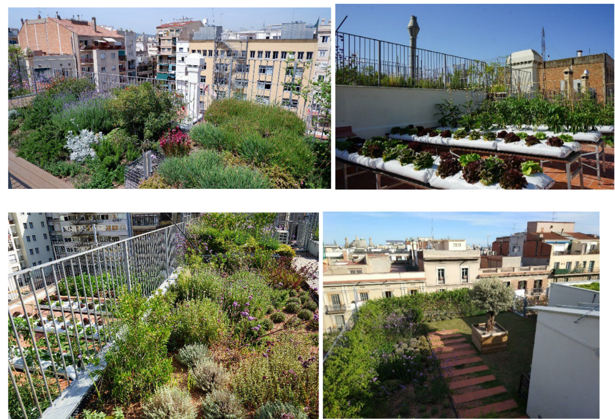
Fig. 9. Semi-intensive green roof located at Pérez-Iborra school, Barcelona.
