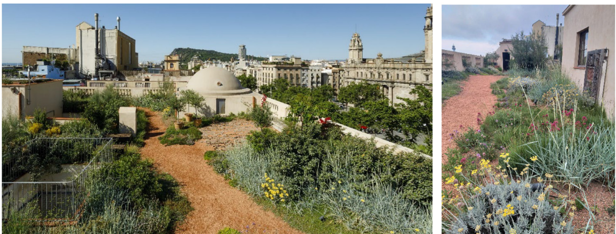
Fig. 1. Example of Building-Integrated Greenery systems in Barcelona. Porxos d'en Xifré Semi-intensive green roof.
