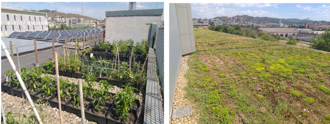
Fig. 3. Example of Building-Integrated Greenery systems in Barcelona. TEBVerd Extensive and urban vegetable garden green roof.
